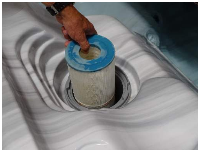
Figure 16. Drop in filter removal
