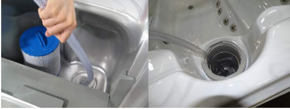
Figure 7. Filling Location in Filter Housing
