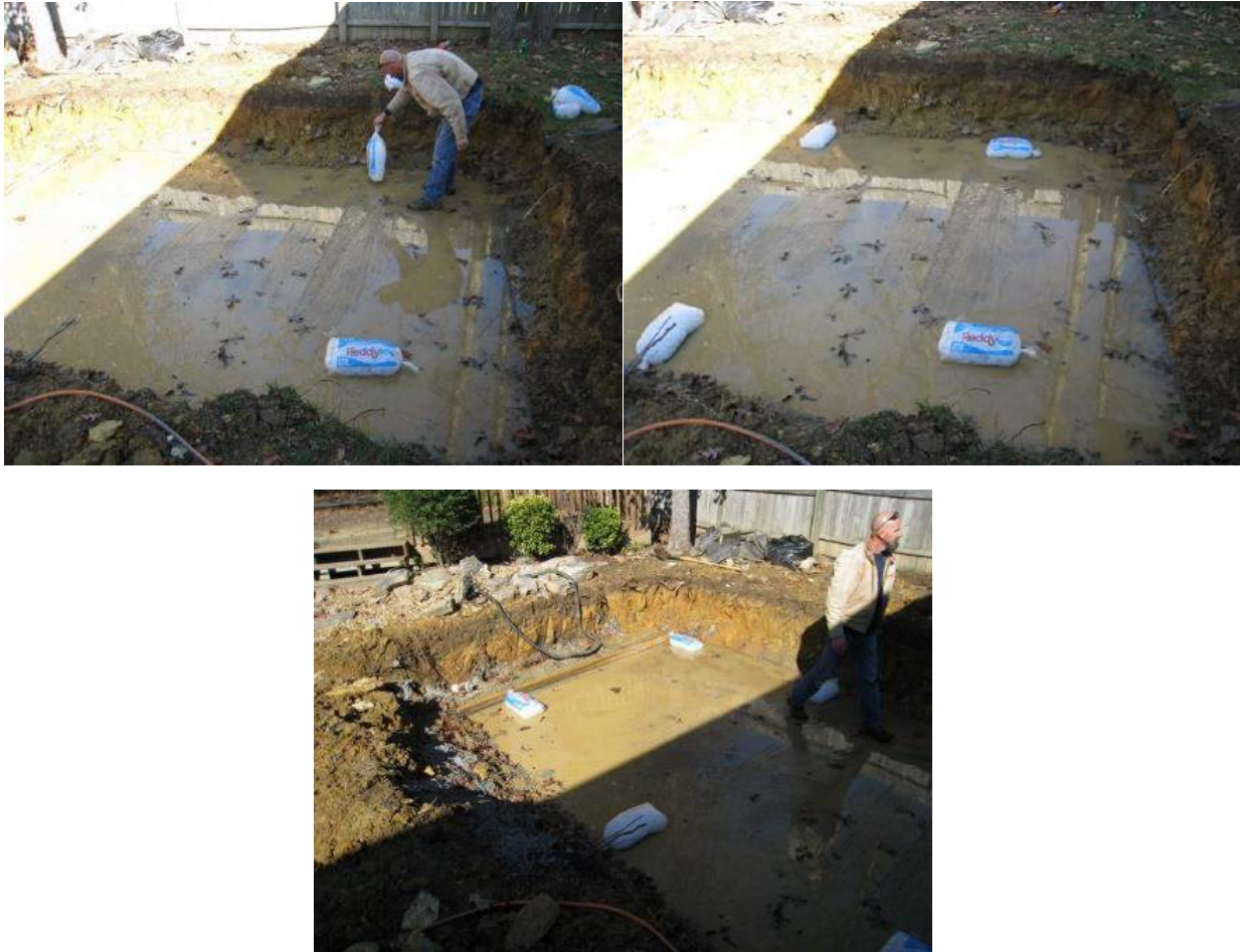
Figure 7. Ice Bag Positioning in Excavation
